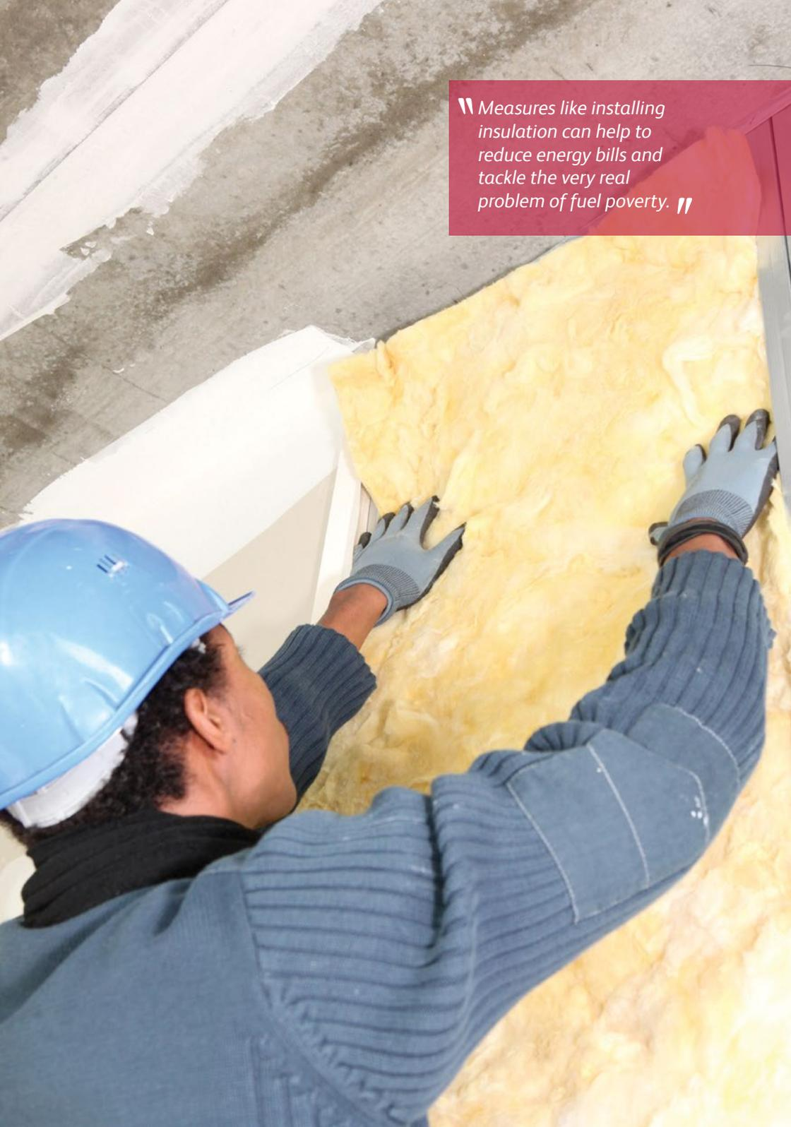
A high-angle photograph of a worker installing insulation. The worker is wearing a blue hard hat, a blue ribbed sweater, and blue work gloves. They are leaning over a wall, carefully placing a large sheet of yellow, fibrous insulation. The wall is partially covered with white insulation, and the floor is made of concrete. The lighting is bright, highlighting the texture of the insulation and the worker's clothing.
